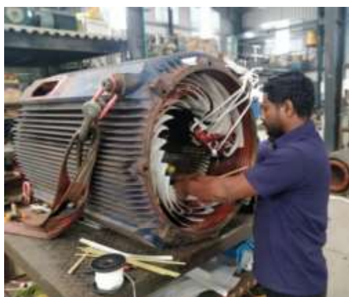
Mechanical stability of the coil
